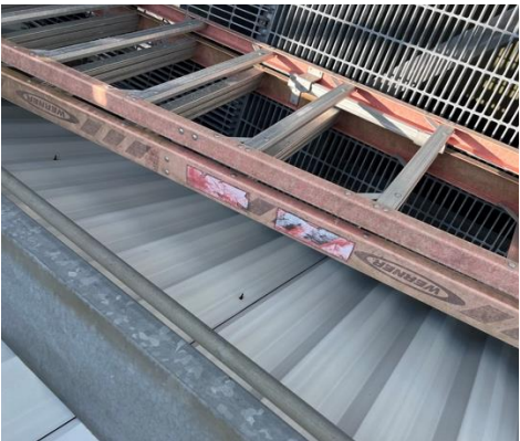
Ladder no inspection tags
