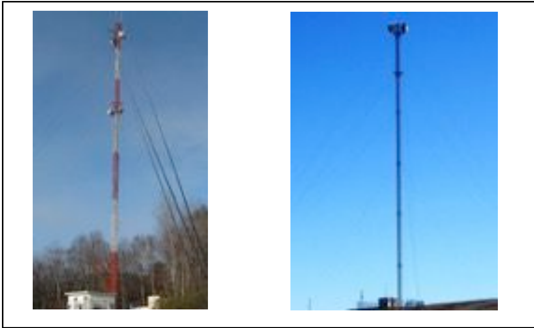
Guyed Lattice Masts
