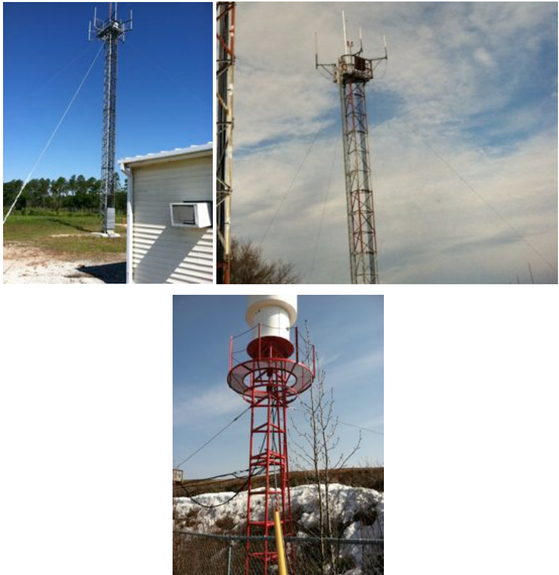
Self-supporting Towers Affixed with Guy Wires
