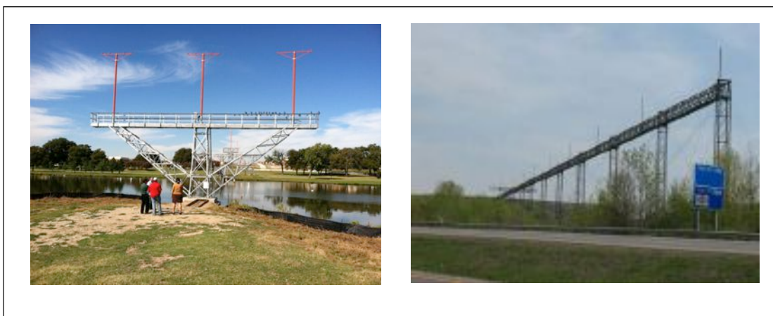
Complex Tower, Mast, and Pole Systems
