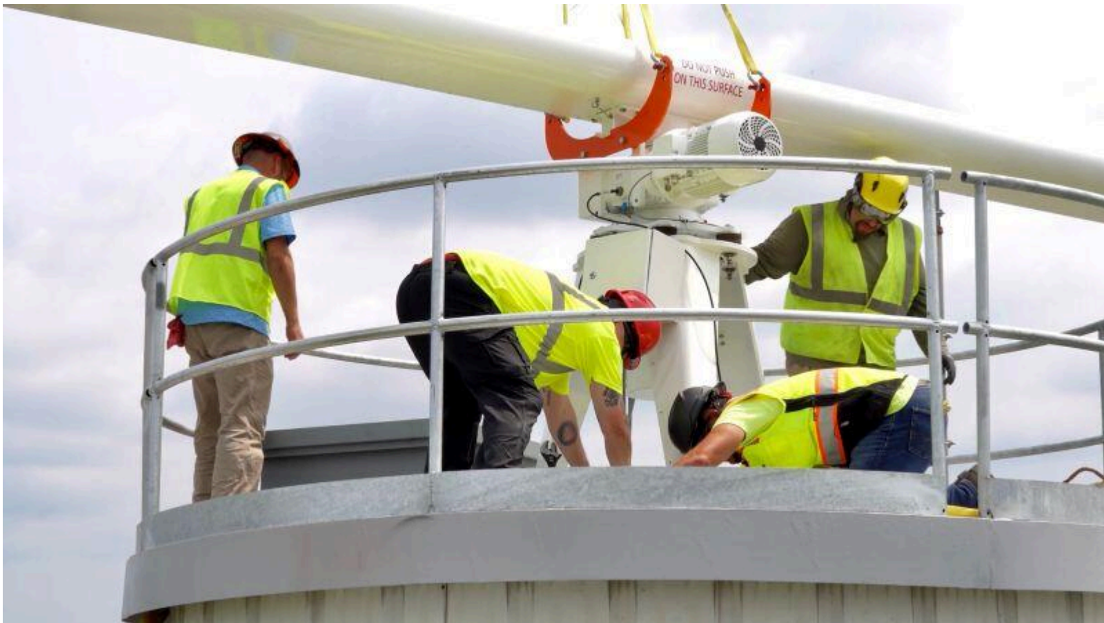
Technicians ready surface movement radar antenna for installation at Ronald Reagan Washington National Airport in August.
